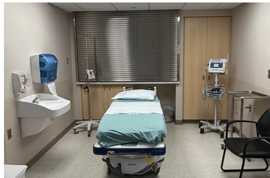
Left Picture: Medical equipment on the wall is exposed providing a threat to the patient and staff.
